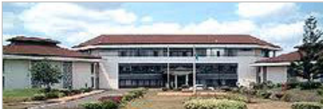
KEMRI Campus at Kisumu
